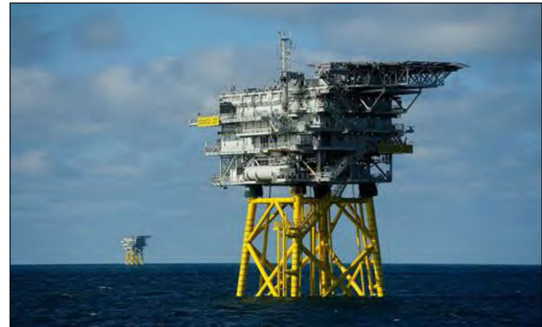
Figure 3.17: Offshore substations at Gode Wind offshore wind farm.
