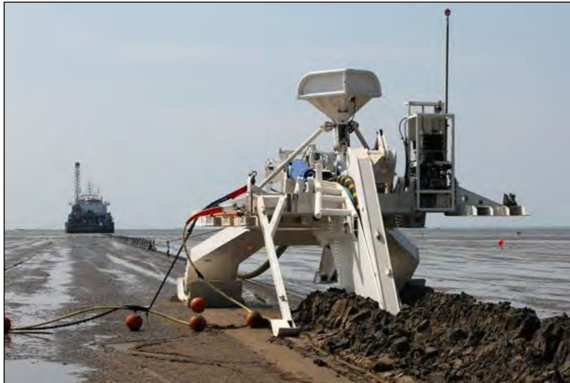
Figure 3.24: Example of a cable plough pulled from an installation vessel.
