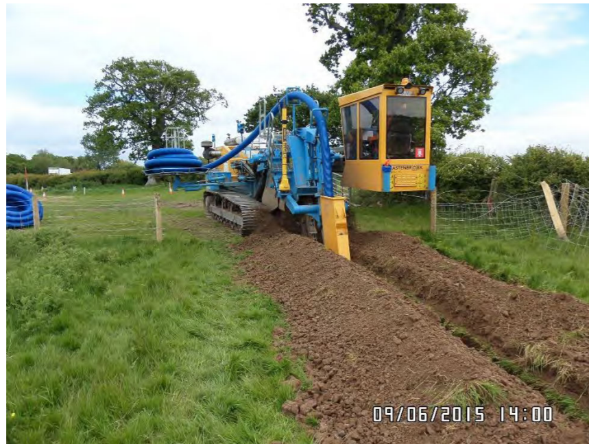
Figure 3.26: An example of a tracked tool used for pre-construction drainage.
