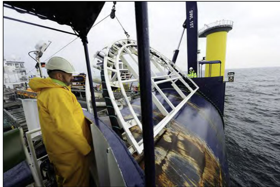
Figure 3.15: Array cable installation at the Gode Wind offshore wind farm.
